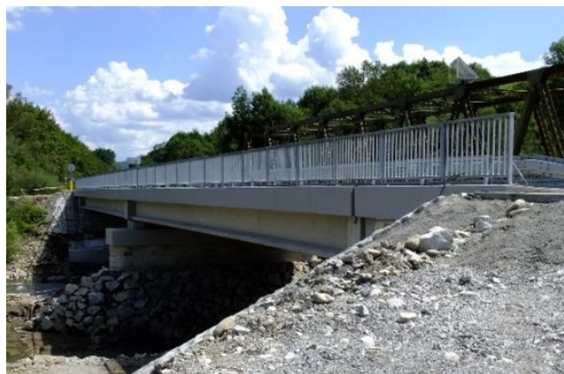
Fig. 8a. View on the rehabilitated structure.
