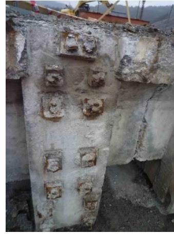
Fig. 5b. Anchorage zone.
